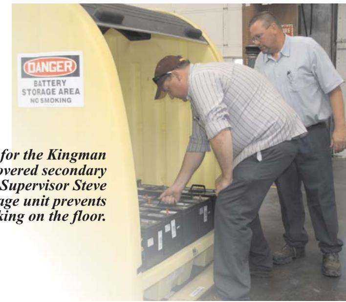
*David Arnold, Jr., parts expeditor for the Kingman shop, removes a battery from the covered secondary containment storage area. Shop Supervisor Steve Carspecken, right, says the storage unit prevents battery acid from potentially leaking on the floor.*
